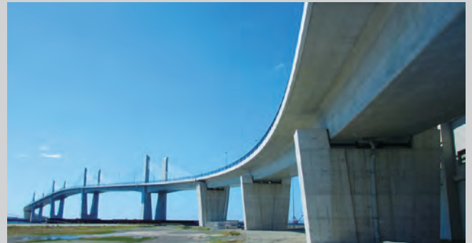
「小名浜マリブリッジ(3号ふ頭部)」PC4径間連続箱桁橋の設計 (土木学会田中賞2018) Onahama marine bridge (No.3 dock), a successive pre-stressed concrete box-girder bridge with four spans
