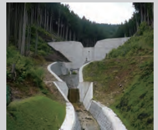
不透過型堰堤 Impermeable type SABO dam
