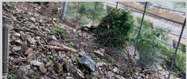
設計した崩壊土砂防止柵により土砂災害を防いだ事例（道路防災点検・防災設計） Example of sediment disaster protection by designed collapse prevention fence (Inspection and design for road disaster prevention)
