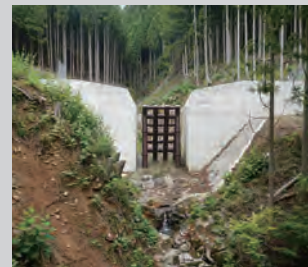
透過型堰堤 Slit type SABO dam
