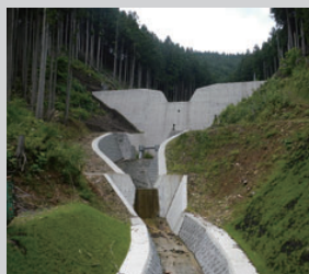
不透過型堰堤 Impermeable type SABO dam
