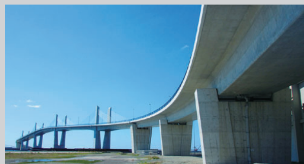
「小名浜マリナブリッジ(3号ふ頭部)」PC4径間連続箱桁橋の設計 (土木学会田中賞2018) Onahama marine bridge (No.3 dock), a successive pre-stressed concrete box-girder bridge with four spans
