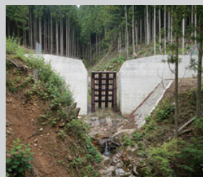
透過型堰堤 Slit type SABO dam
